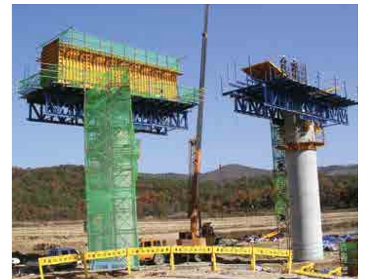
+ 1st section of Donghae Expressway - Korea
