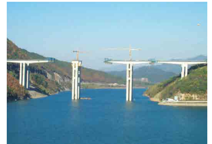
+ Shindanyang Large Bridge - Korea
