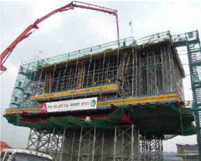
+ Gyeongin Ara Waterway Section 6 - Korea
