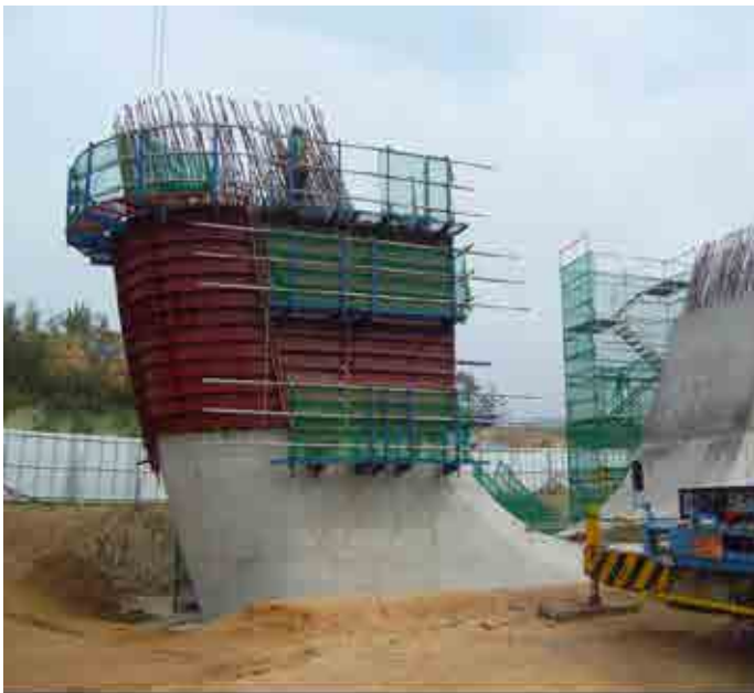
+ 4th Geumgang Bridge - Korea
