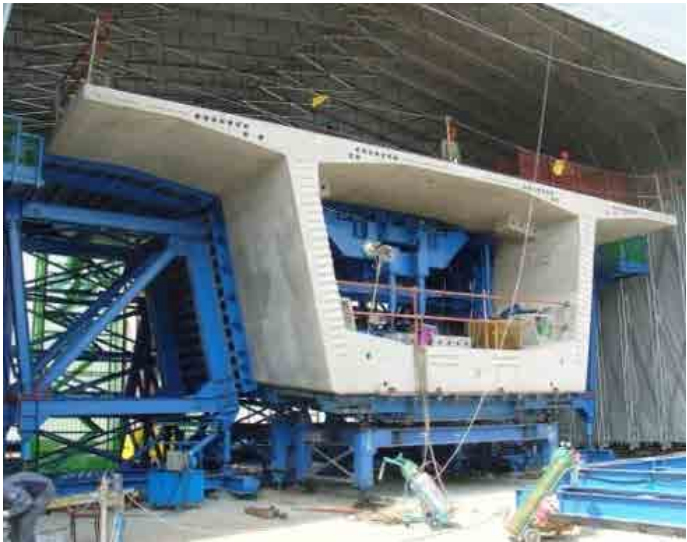
+ Incheon Grand Bridge - Korea
