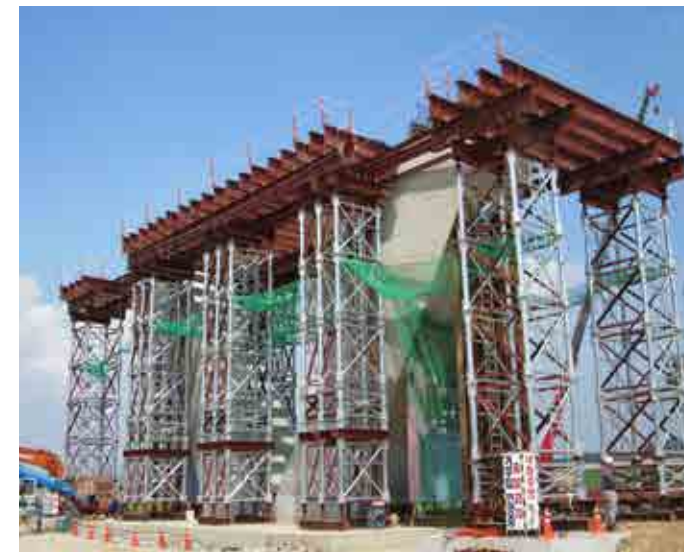
+ Miho stream Bridge - Korea
